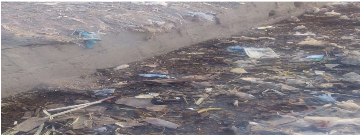
Plate 4: Disposal of wastes along and into drainage systems
