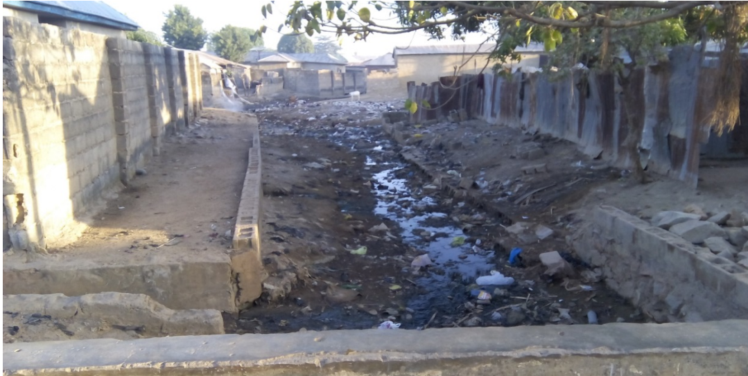
Plate I: Dump in drainage in Chanchaga.
