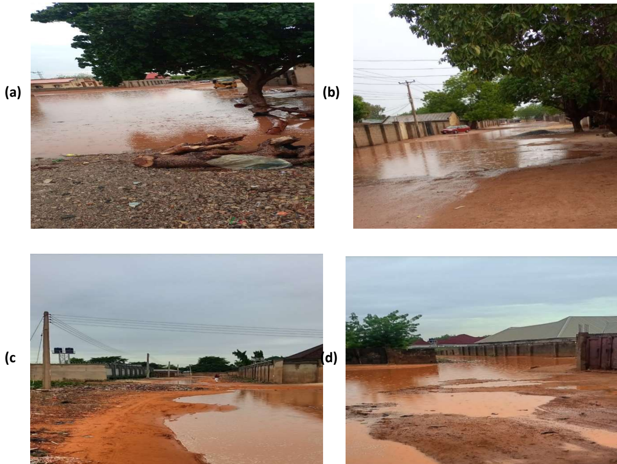
(a) Flooded street with silted drainages (b) Flooded street with no drainages (c) Street overtaken by household solid waste and impeded surface runoff (d) Flooded houses after rains
